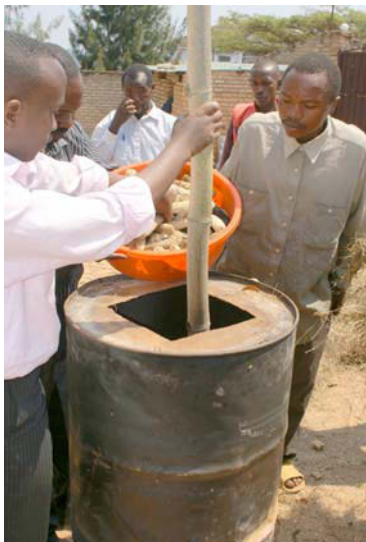
Figure 7: Fill the drum with a central chimney Photo credit: Fuel from the Fields
