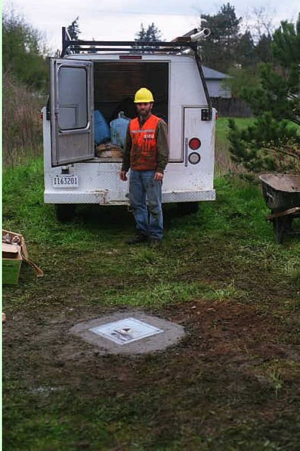
Flush-mounted well
